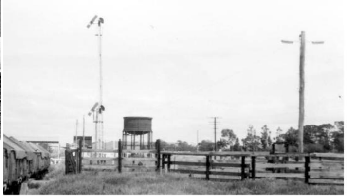
Photograph of the 1887 Water Tower also in the foreground of the photograph are the livestock yard, wheat trucks on the left and semaphore signals indicating that a train is coming.
